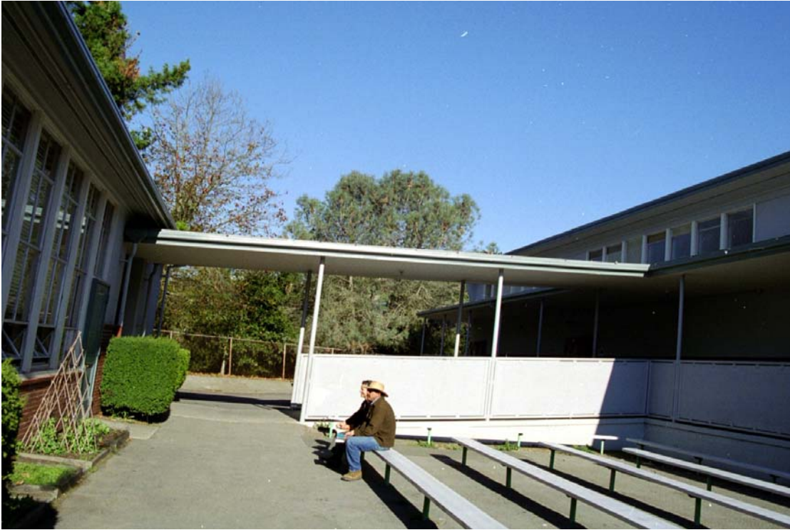
Figure 9: Covered Walkway Between Buildings
