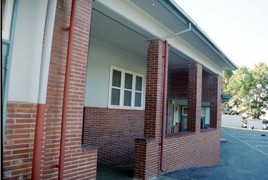
Figure 8: Main Building Northwest Exterior Corridor
