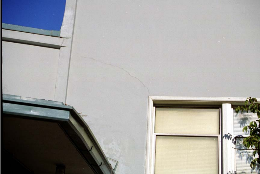
Figure 7: Main Building – Plaster Cracks
