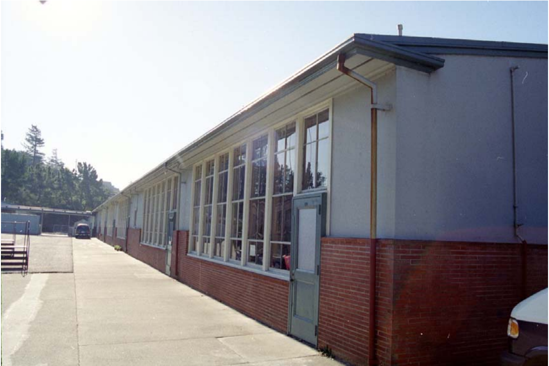
Figure 3: Classrooms East longitudinal Walls
