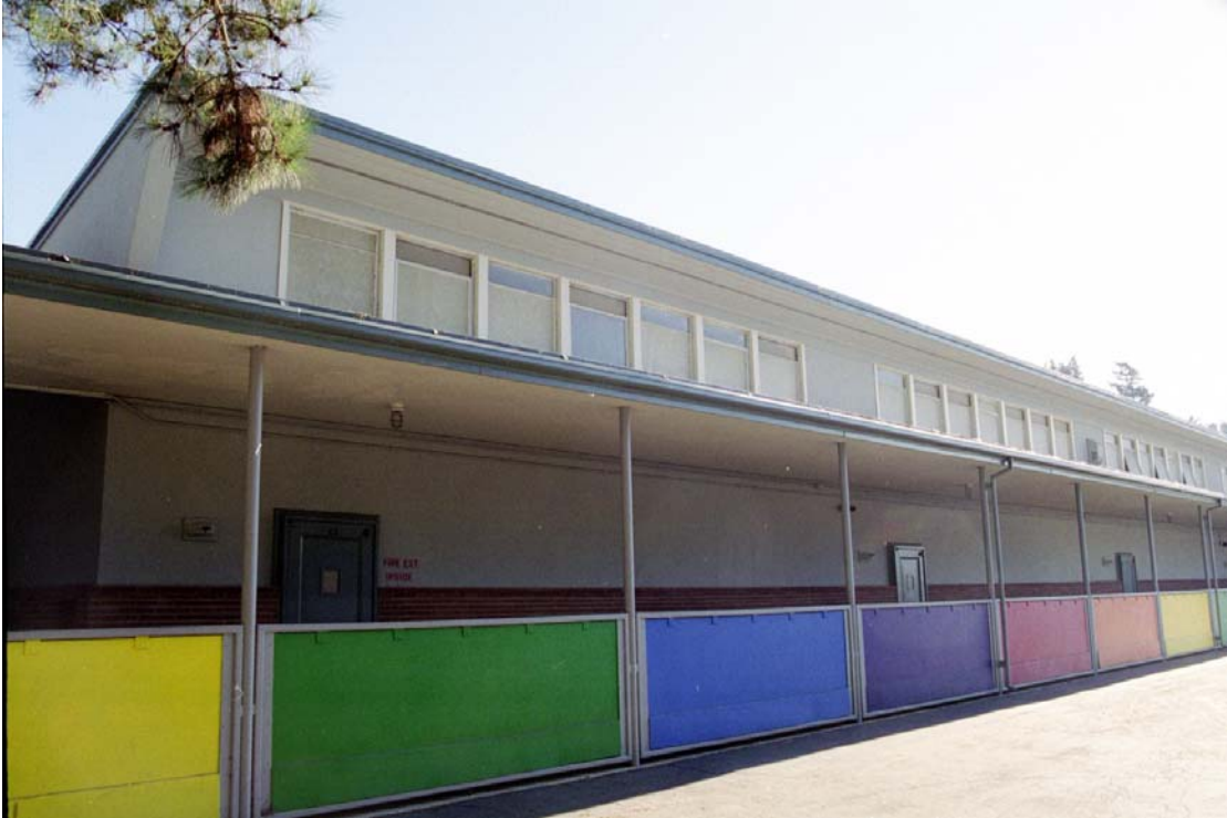
Figure 4: Classrooms with Clearstory Windows, West Longitudinal Walls
